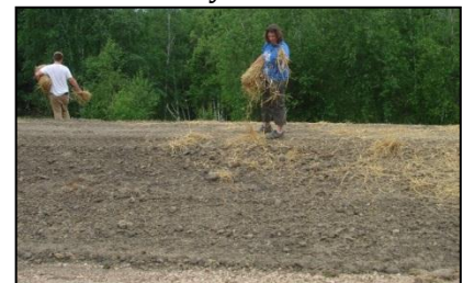
Above: Visual berm being constructed. Below: Laying seed and hay on visual berm.
