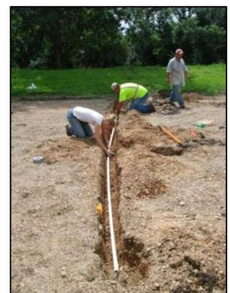
Above (left): View of a lysimeter in a 3' deep hole. Above (middle): A UMN graduate student pours the sealant into the lysimeter hole. Above (right): SET staff place lysimeter tubes in PVC pipe for added protection.
